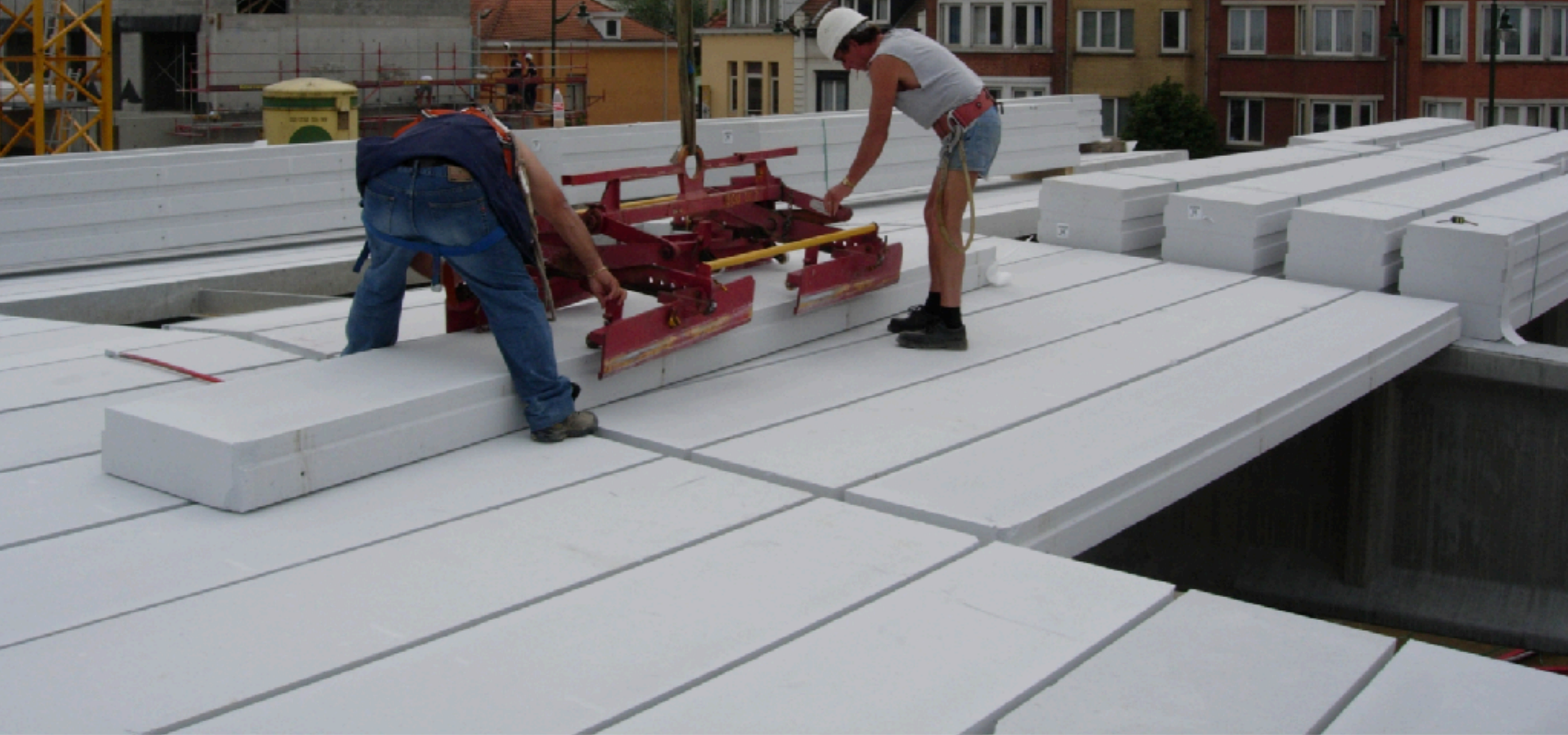
The modular building systems allows a floor to be installed within hours
